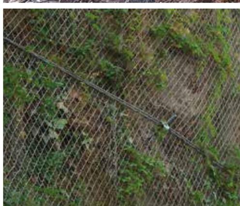
The wire used to manufacture **3STutor®Plus** mesh is specially produced and assures a higher protection against corrosion, having a Zinc-Aluminium coating class A or, on demand, even higher.
